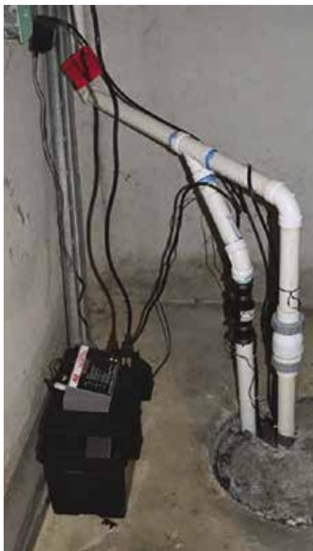
**Safety tip: Make sure a ground fault circuit interrupter (GFCI) outlet is used to plug the sump pump into.**
