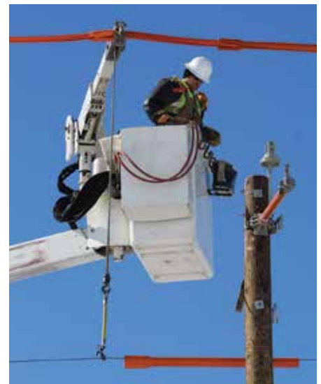
Lineworker Lee upgrading infrastructure along County Road D.
