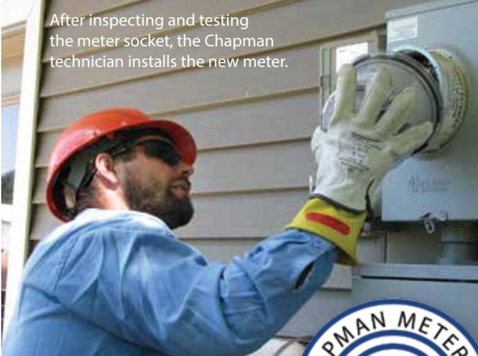
After inspecting and testing the meter socket, the Chapman technician installs the new meter.
